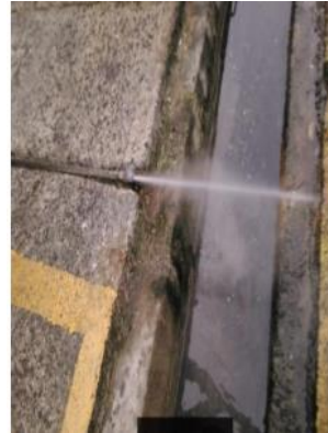
Water leakage
